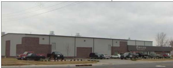
Completed! Empire Sheet Metal's new facility
