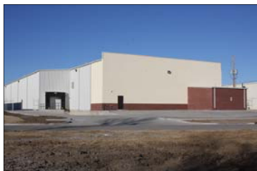
Completed! New facility for Broken Arrow Electric Supply
