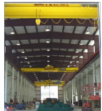
Completed! New crane building for Cust-O-Fab in Sand Springs.
