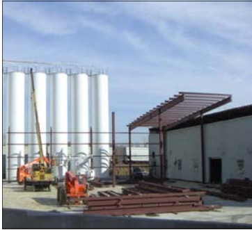
Under Construction! New Sigma Stretch Film facility.
